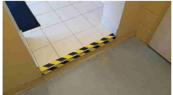
Sample: Floor level Transition Location: Stair No. 1
