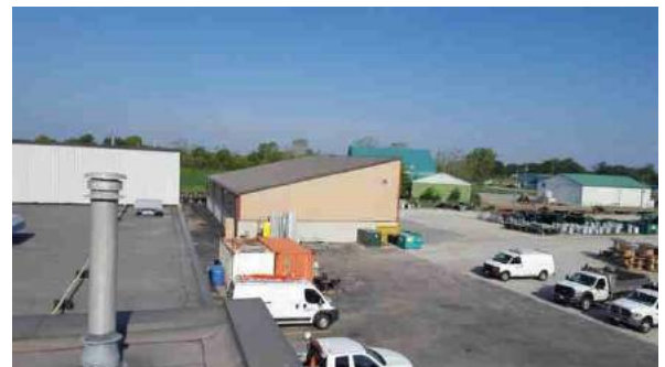
Pitched metal roof Location: Works Garage
