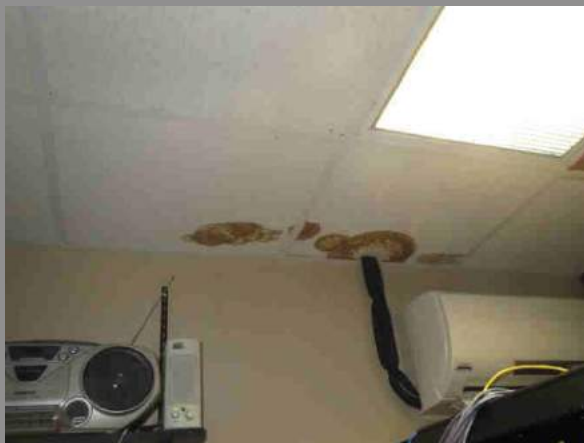
Sample- Ceiling tile damaged (condensation from HVAC Equipment) Location: Second Floor Communication Room
