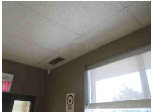
Repair: Water damaged ceiling tiles Location: Second Floor
