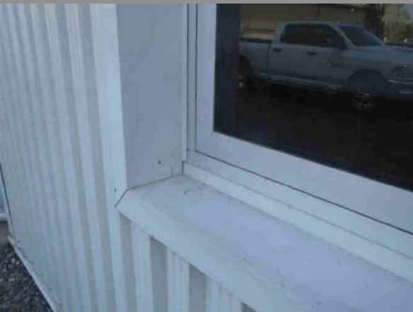
Sample: Window and Flashing in good condition Location: west Wall of Main Building
