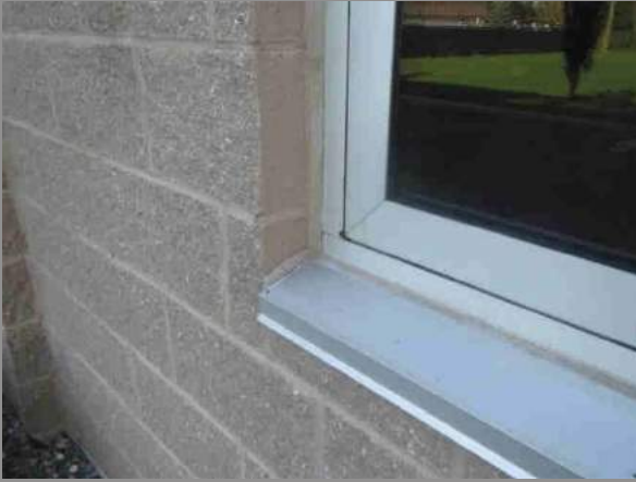
Sample: Window and Caulking in Good shape Location: Southwest Wall
