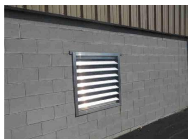
Sample: Conc. Block, Louver Location: Works Garage
