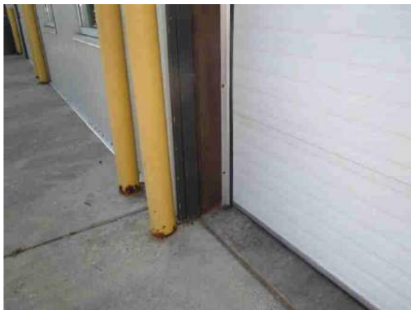
Repair: Rust at overhead doors Location: Inventory door (No. 5)
