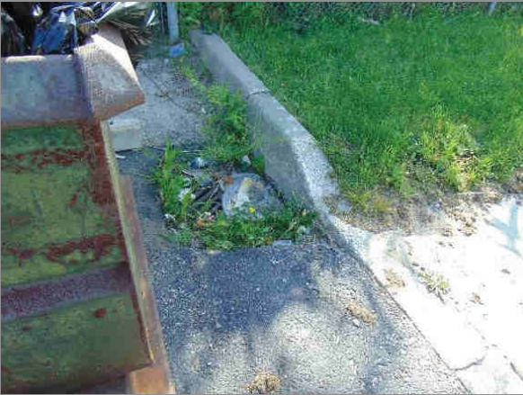
Catch Basin Settlement Location: North Service Area
