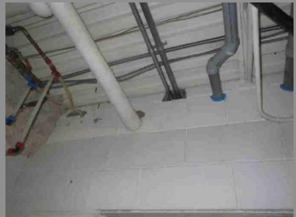
Penetration not fire caulked. Location: Mechanical Room
