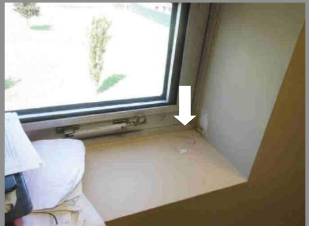
Repair: Window Leaking Location: Second Floor Office
