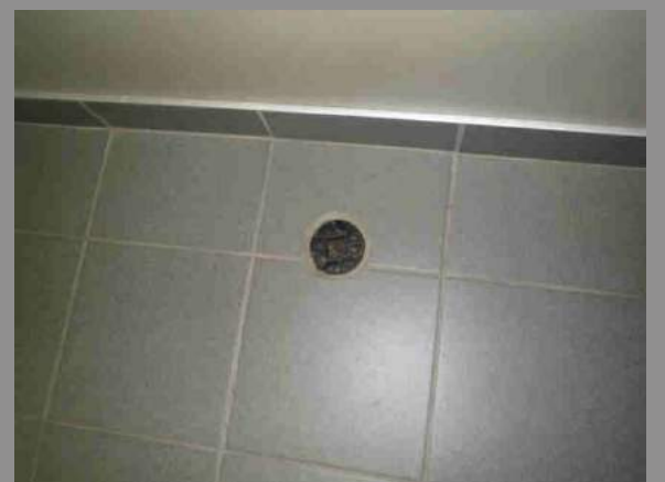
Sample: Cleanout missing cap – trip hazard Location: First Floor Kitchen
