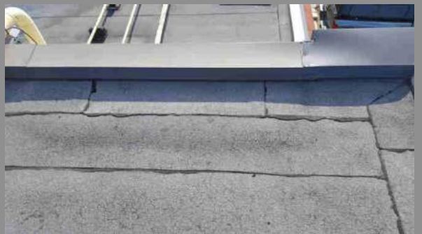
Roof starting to Bubble Location: One Storey Office Area - By Training Room
