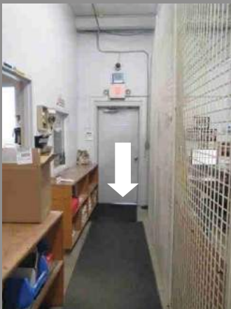
Repair: Weatherstripping missing Location: Shipping & Receiving
