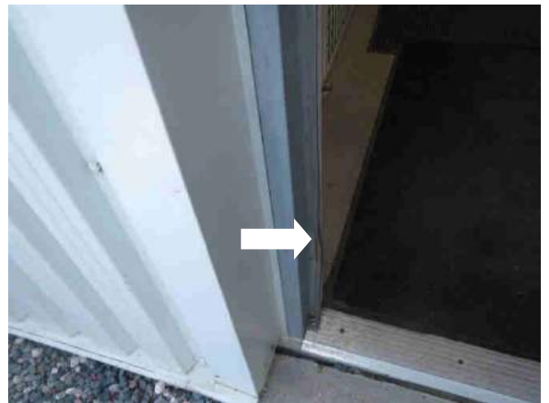
Repair: Weatherstripping Damaged Location: Shipping & Receiving
