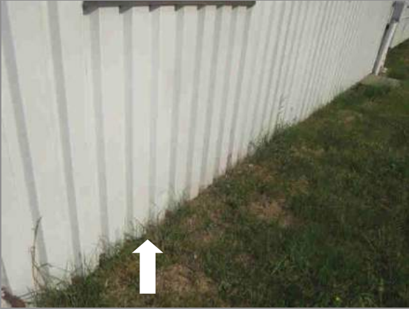
Repair: Grade over Metal Siding Location: Outside Training Room
