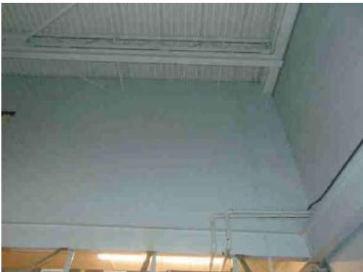
Possible Lateral stability issue Location: Storage Area
