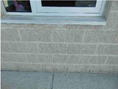
Cracking in Exterior Facade Location: South Wall
