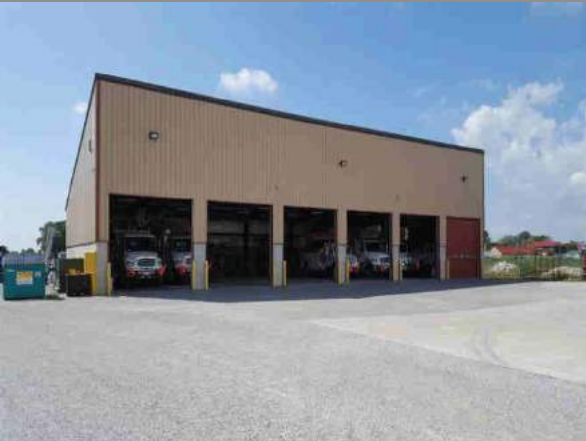
Front View of Works Garage Location: Works Garage
