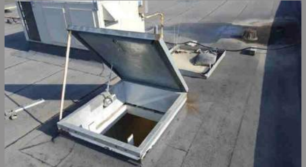
Roof Hatch Location: Over second Storey Office
