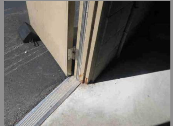
Repair: Door Frame rusting – frame does not fit masonry opening Location: Works Garage
