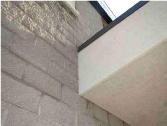
Sample: EFIS and Masonry Joint Location: Main Entrance
