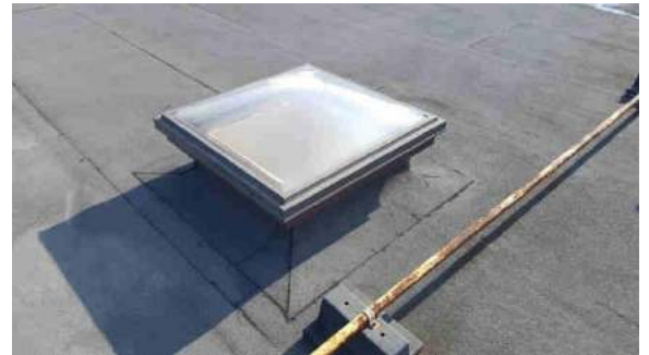
Skylight Location: Over Second Floor Office
