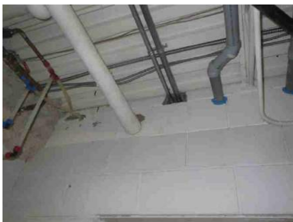
Sample: Concrete slab in good condition Location: Truck Bay
