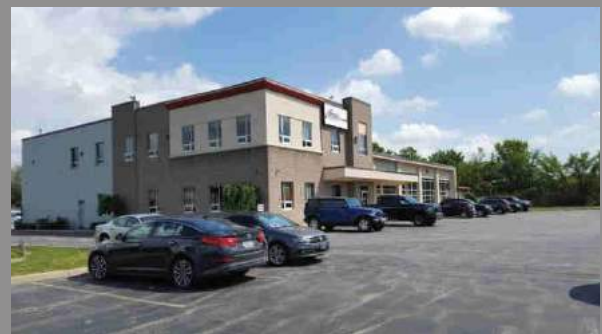
Sample: Metal Siding, EFIS and Masonry Facade Location: Looking at Main Entrance
