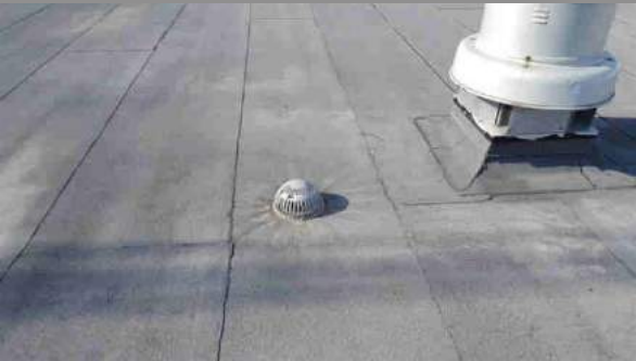
Exhaust fan c/w new seals on curbing Location: Over First Floor Office Area
