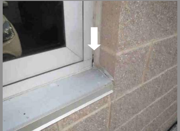
Repair: Caulking failing Location: Southwest Wall
