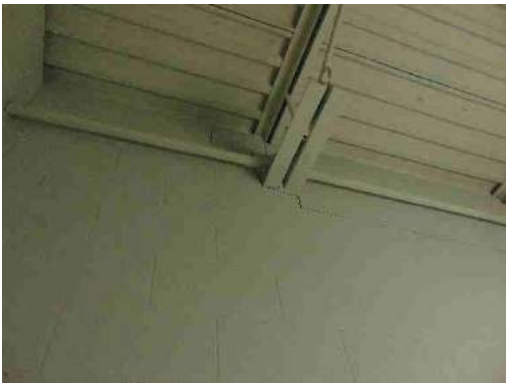
Cracking in Wall Location: North Stairwell
