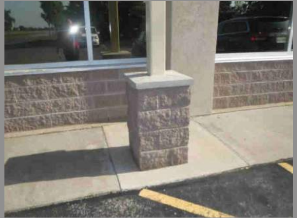
Sample: Masonry Pier | Sidewalk Location: South Wall
