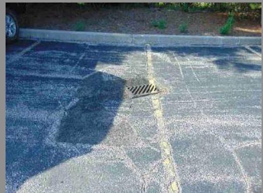
Catch Basin Location: South Parking Area
