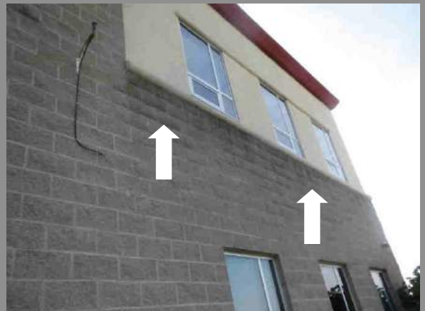
Monitor: Possible moisture intrusion Location: Southwest Wall
