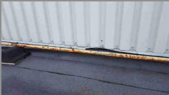
Rusted Counter Flashing at High Wall Transition Location: At Meter Shop – Office
