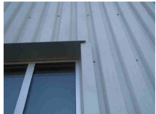
Sample Metal Siding Location: West Wall
