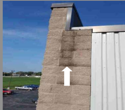
Monitor: Possible moisture intrusion Location: Front Entrance
