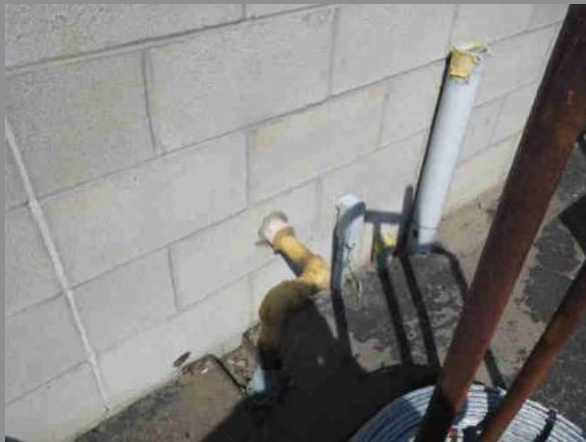
Sample: Penetration sealed Location: Works Garage
