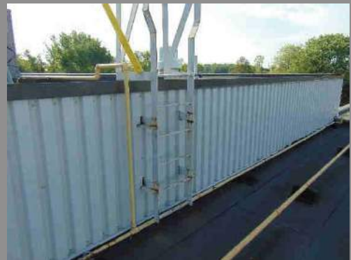
Typical Roof Ladder Location: Roof
